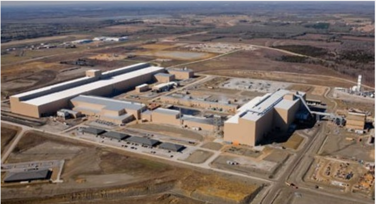
Figure S1: Grid-Tied Energy Storage in the Southeast
