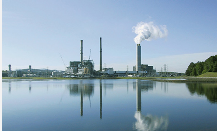
Figure S5: Asheville Energy Plant [83]
